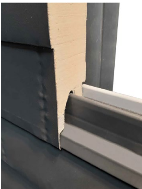
| Panel joint detail
