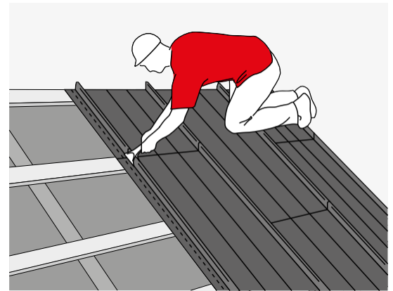
FIG. 30. CRIMPING THE PANEL LOCKS ALONG OVERLAPS
