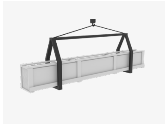
FIG. 5. UNLOADING THE ROOF PANELS
