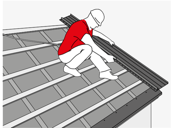
FIG. 16. LAYING THE ROOF PANELS
